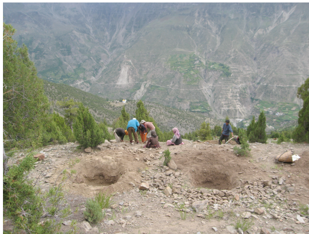
Plate 1: Community Participation for construction of Snow Pits in Sakling, Himachal Pradesh, India
